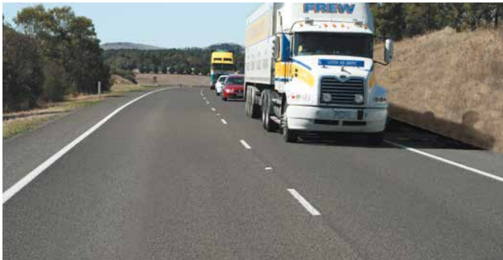
10mm OLEXOBIT SP reseal sprayed at 1.2 to 1.4 L/m 2 on the Calder Highway near the 52km post on the Melbourne outbound lanes (near Gisborne) in Victoria.
